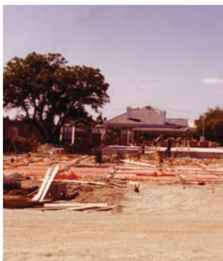
Roselin Court under construction
