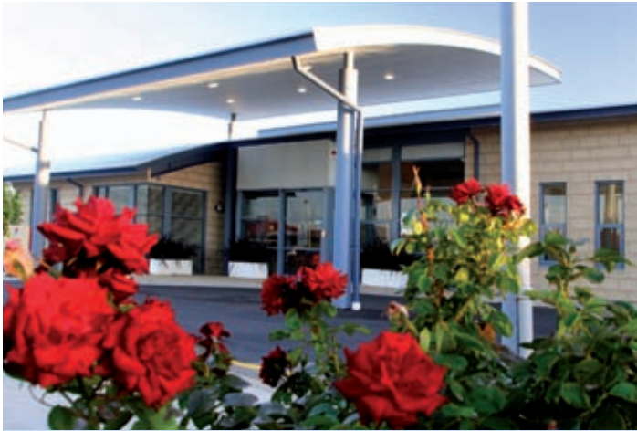
Aldinga Beach Court, a stylish new residential care facility
